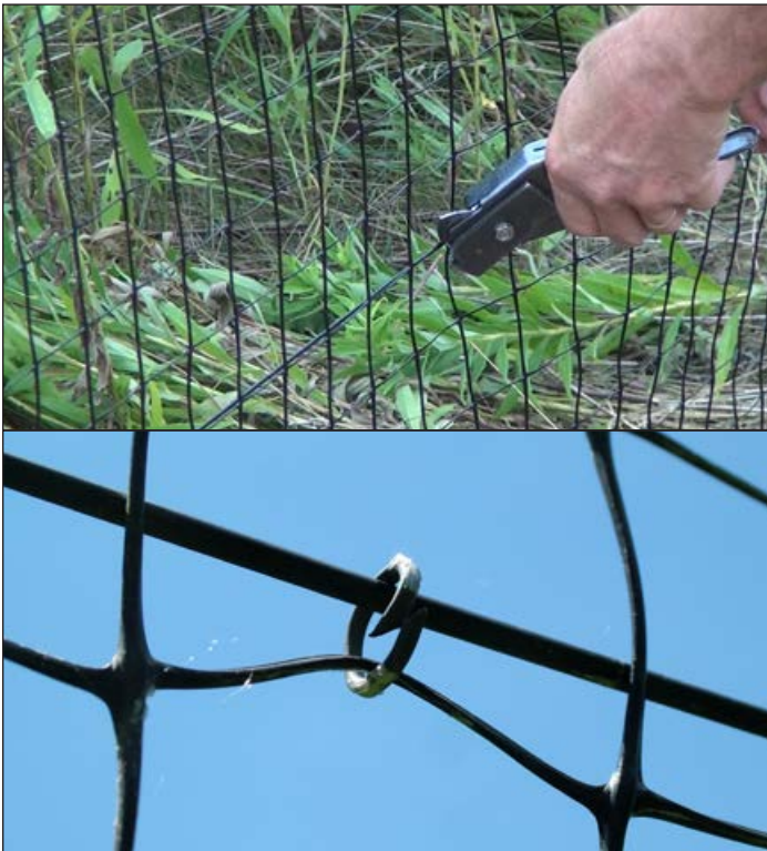
Figure 10. Use a hog-ring plier to attach the mesh to the monoline.
