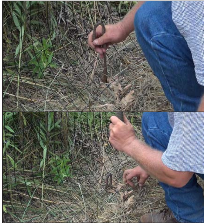
Figure 11. Stake the bottom of the fence once or twice between posts to reduce the pulling effects of the wind and to prevent deer from crawling under the fence.
