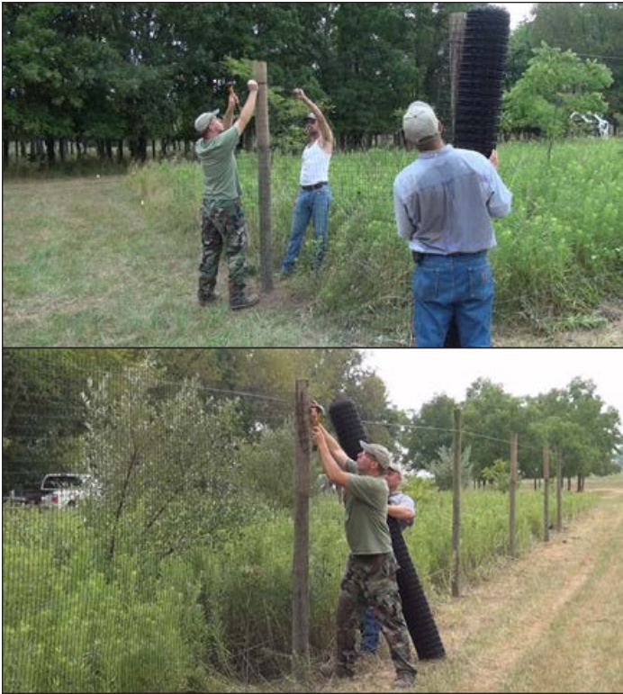
Figure 9. Position and nail the plastic mesh to the posts, being sure one square or about 2 inches of mesh are above the top monoline and 4 or 6 inches overlap the ground.
