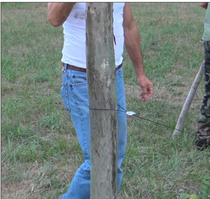
Figure 7. Tension and trim the middle monoline.
