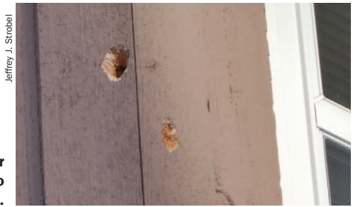
Woodpecker damage to house siding.
