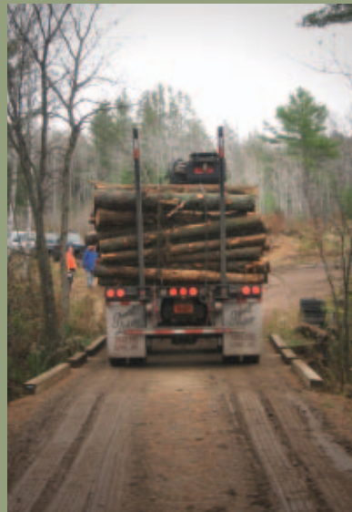
This temporary bridge can support fully loaded logging trucks.
