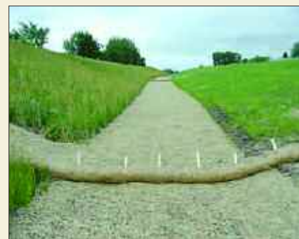
ABOVE: Temporary ditch check with sediment log
