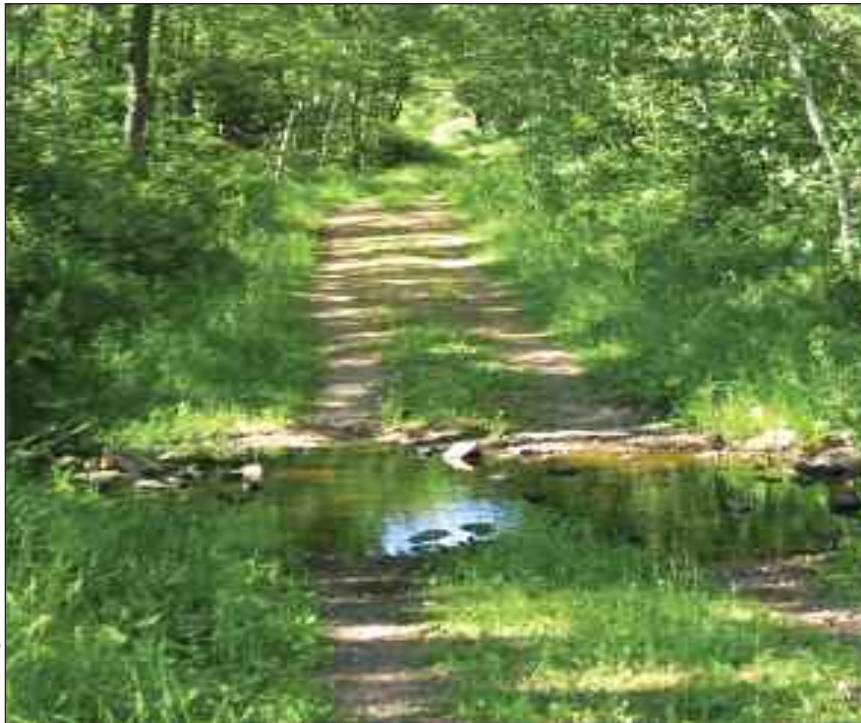
ABOVE: Fords are best suited to shallow streams with a firm rock or gravel streambed.
