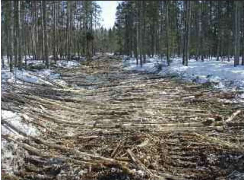
ABOVE: Temporary wetland crossing using slash
