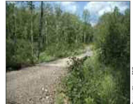
ABOVE: Gravel approaches to a stream crossing
