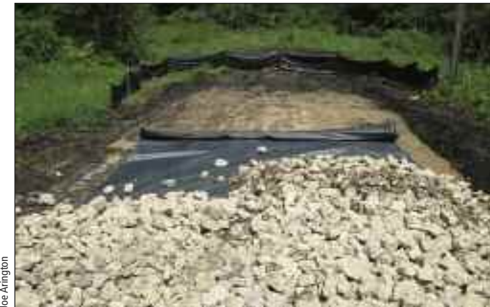
LEFT: Permanent wetland crossing with geotextile
