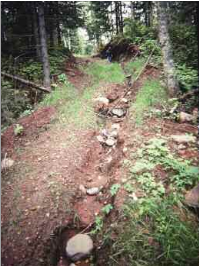
ABOVE: Graveling steep slopes can help to prevent erosion
