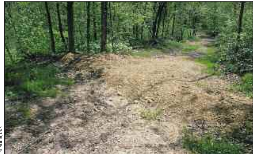
ABOVE: Broad-based dips allow traffic while diverting runoff into the forest
