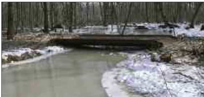
LEFT: Installing temporary stream crossings like this portable bridge, requires a permit from the DNR.
